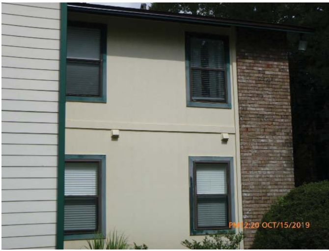
#7 - Opening Protection - None
