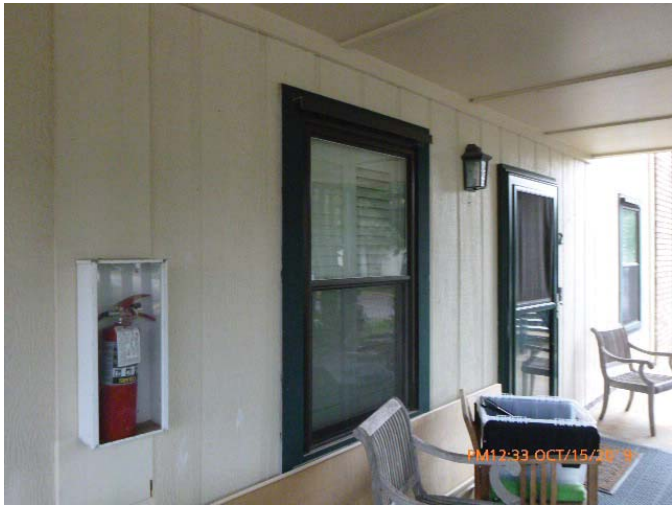
#7 - Opening Protection - None
