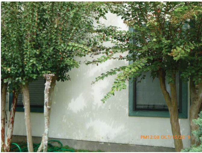
#7 - Opening Protection - None
