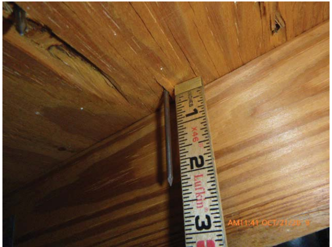
#3 - Roof Deck Attachment - 8d Nail
