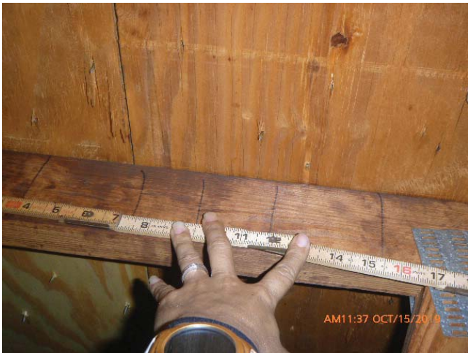
#3 - RDA - 6" or Less Nail Spacing in Field
