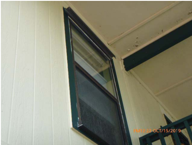
#7 - Opening Protection - Tracks for Shutters
