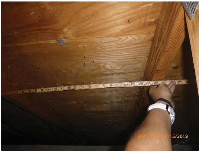
#3 - RDA - Rafter Spacing 24" or Less
