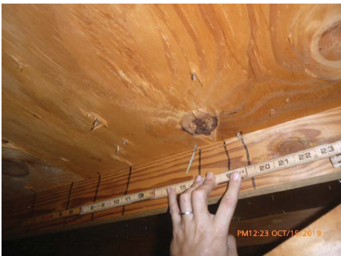
#3 - RDA - 6" or Less Nail Spacing in Field
