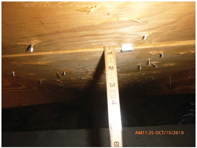
#3 - RDA - Sheathing Thickness 7/16" or Greater
