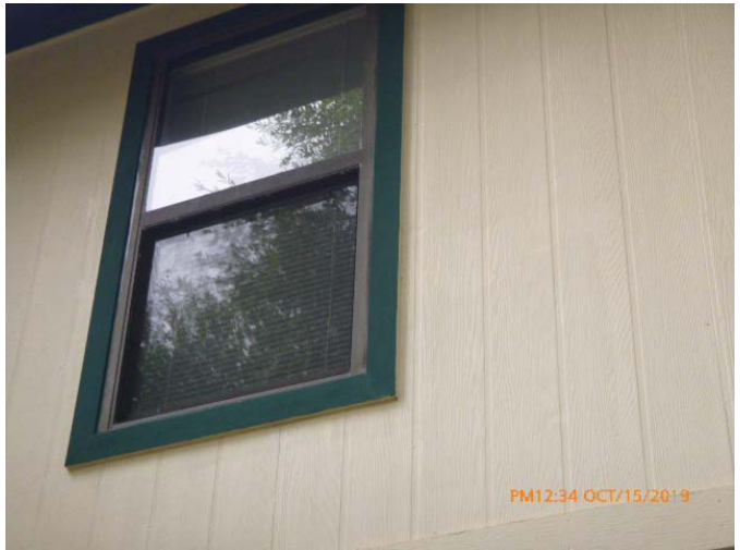
#7 - Opening Protection - None
