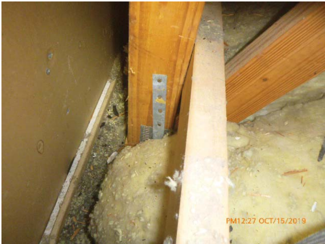
#4 - Roof to Wall Attachment - Hurricane Clips
