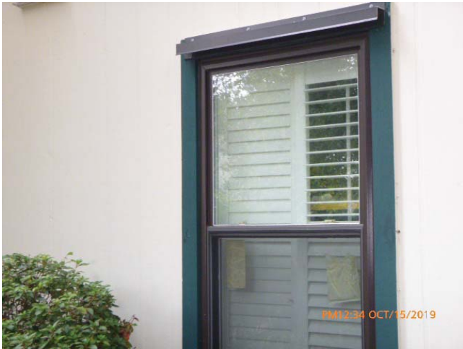
#7 - Opening Protection - None
