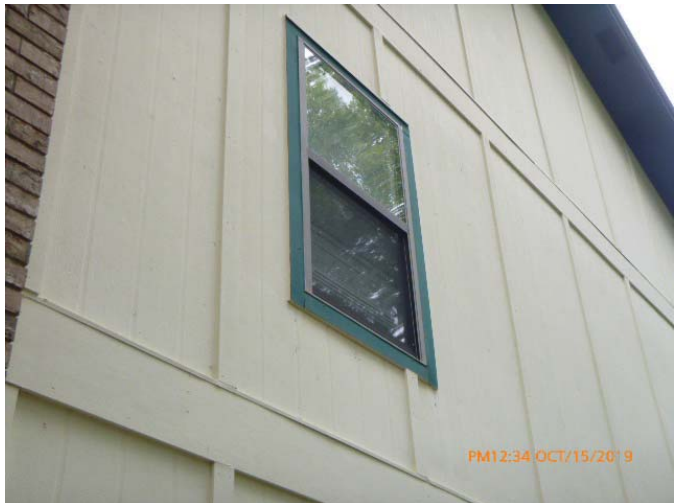
#7 - Opening Protection - None
