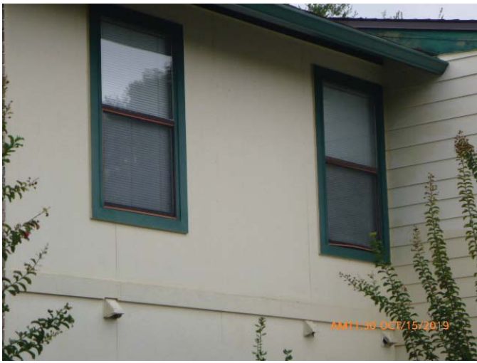
#7 - Opening Protection - None
