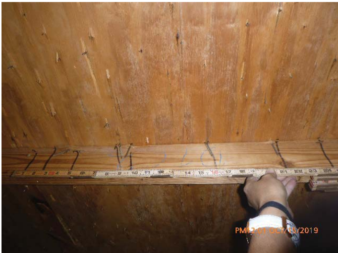
#3 - RDA - 6" or Less Nail Spacing in Field
