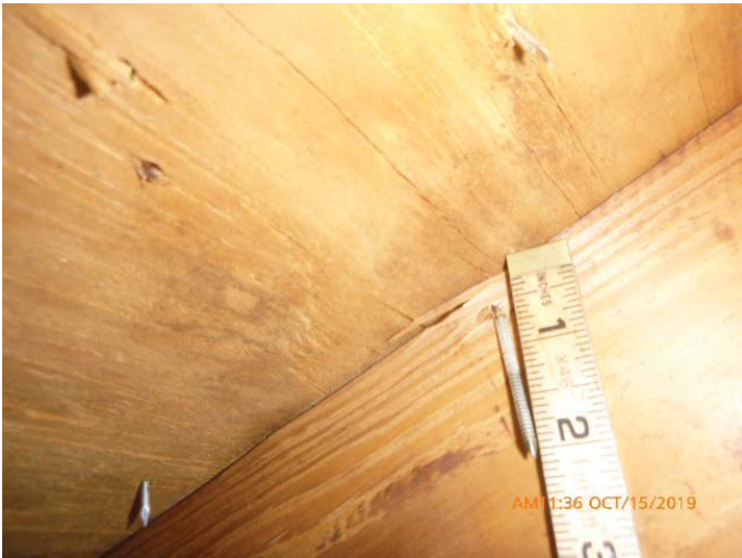
#3 - Roof Deck Attachment - 8d Nail
