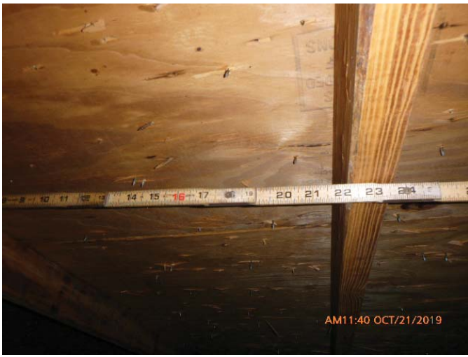
#3 - RDA - Rafter Spacing 24" or Less
