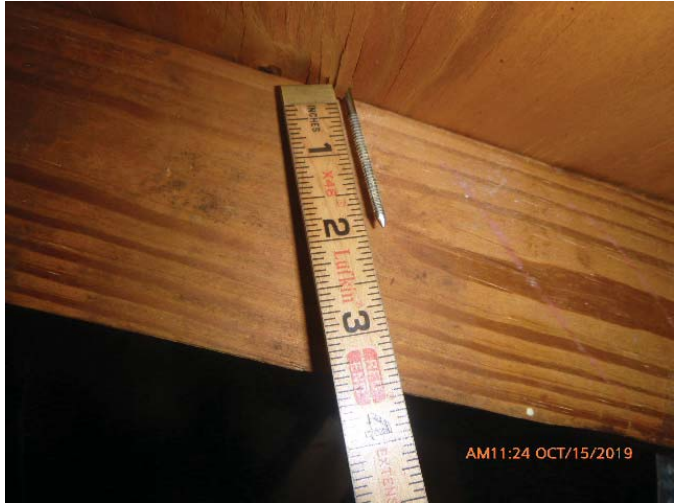
#3 - Roof Deck Attachment - 8d Nail
