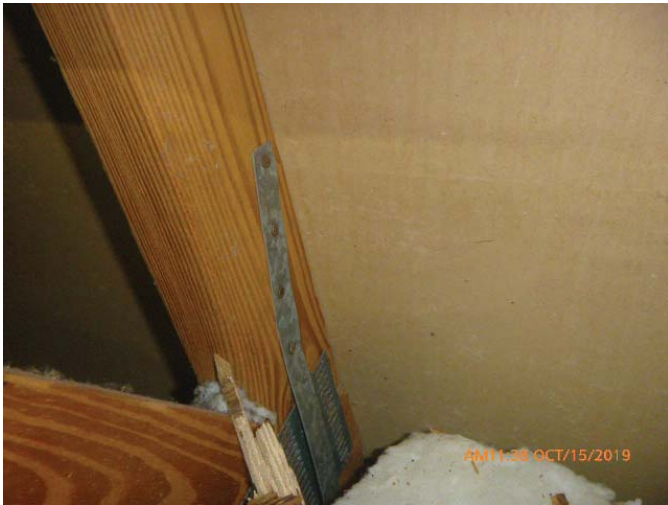
#4 - Roof to Wall Attachment - Hurricane Clips
