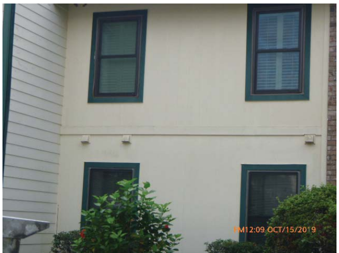
#7 - Opening Protection - None
