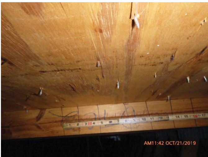
#3 - RDA - 6" or Less Nail Spacing in Field
