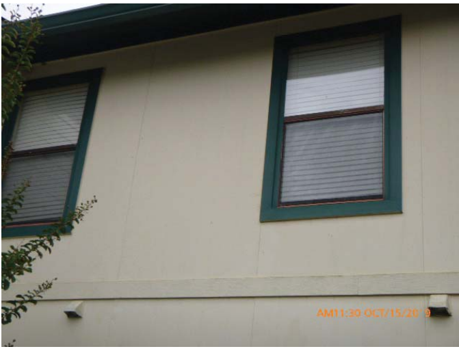
#7 - Opening Protection - None
