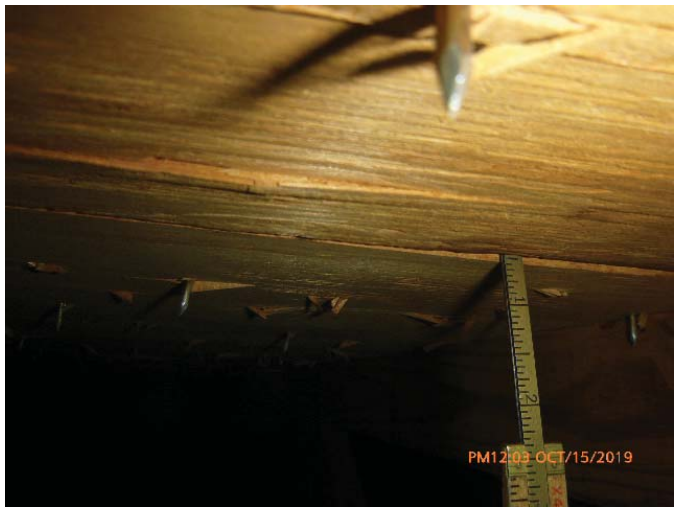
#3 - RDA - Sheathing Thickness 7/16" or Greater
