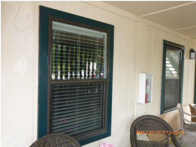
#7 - Opening Protection - None
