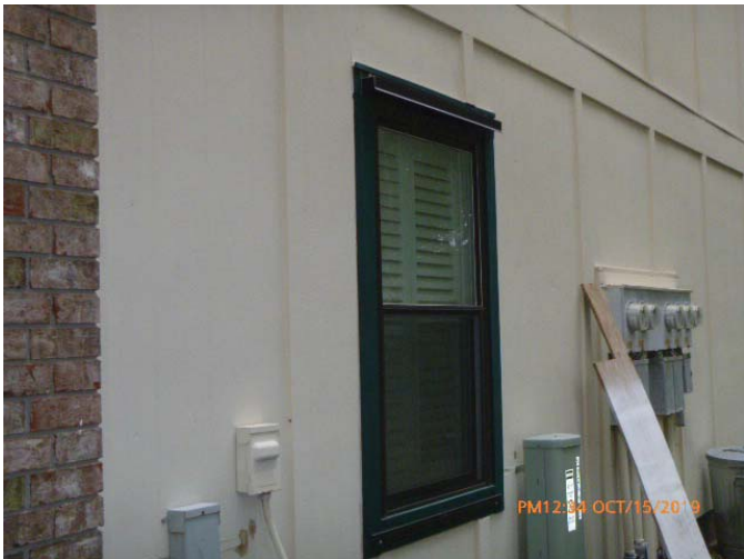
#7 - Opening Protection - None
