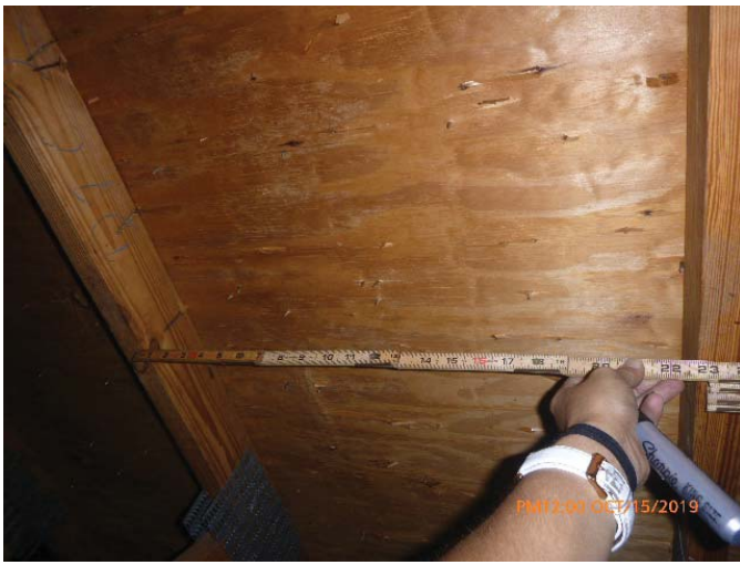
#3 - RDA - Rafter Spacing 24" or Less
