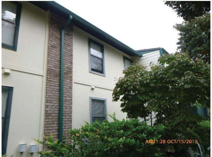
#7 - Opening Protection - None
