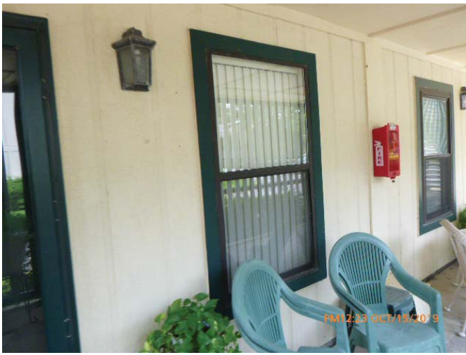
#7 - Opening Protection - None
