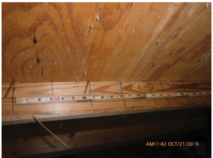
#3 - RDA - 6" or Less Nail Spacing in Field
