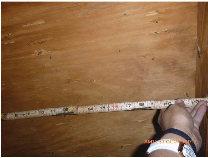
#3 - RDA - Rafter Spacing 24" or Less
