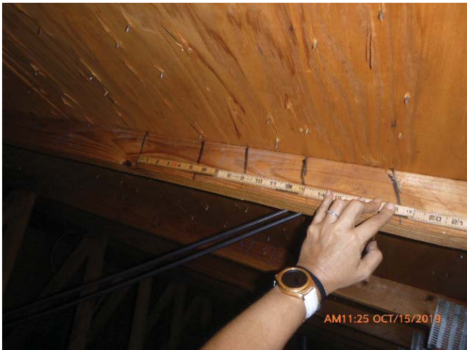
#3 - RDA - 6" or Less Nail Spacing in Field
