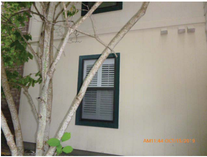
#7 - Opening Protection - None
