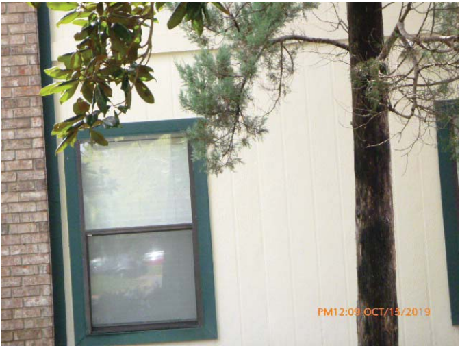
#7 - Opening Protection - None
