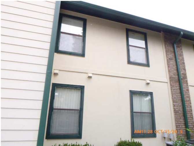
#7 - Opening Protection - None
