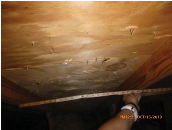
#3 - RDA - Rafter Spacing 24" or Less
