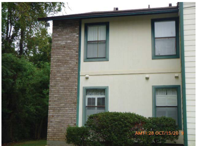
#7 - Opening Protection - None
