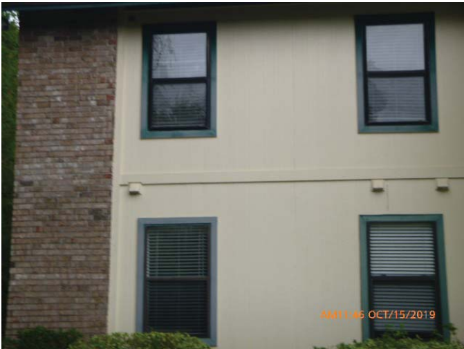
#7 - Opening Protection - None
