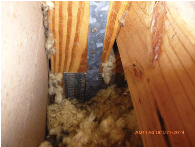
#4 - Roof to Wall Attachment - Hurricane Clips
