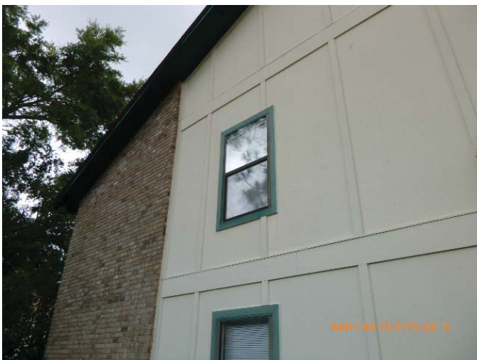
#7 - Opening Protection - None
