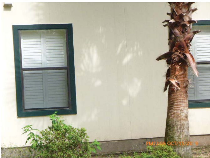
#7 - Opening Protection - None
