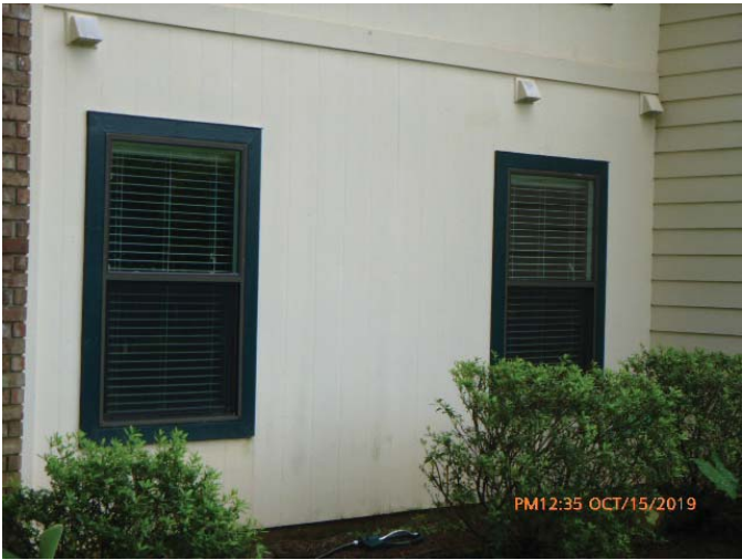
#7 - Opening Protection - None
