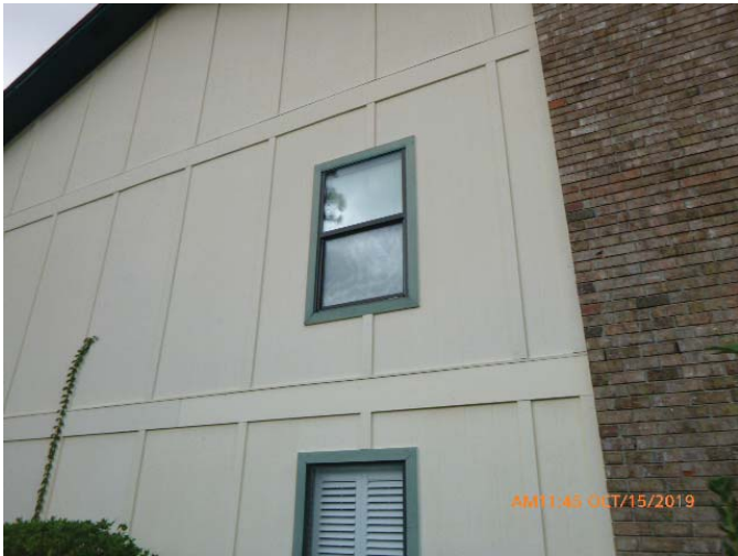
#7 - Opening Protection - None
