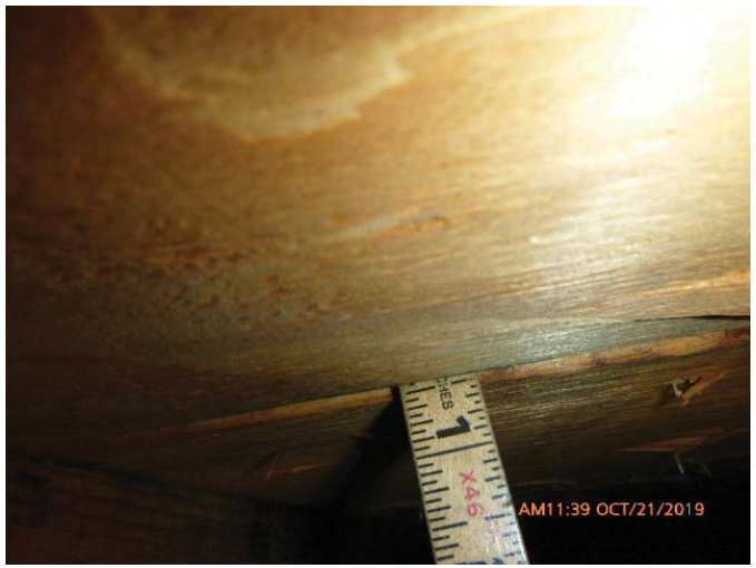
#3 - RDA - Sheathing Thickness 7/16" or Greater
