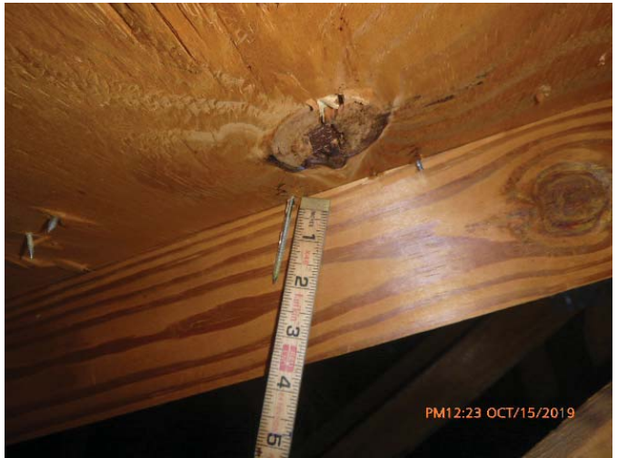
#3 - Roof Deck Attachment - 8d Nail
