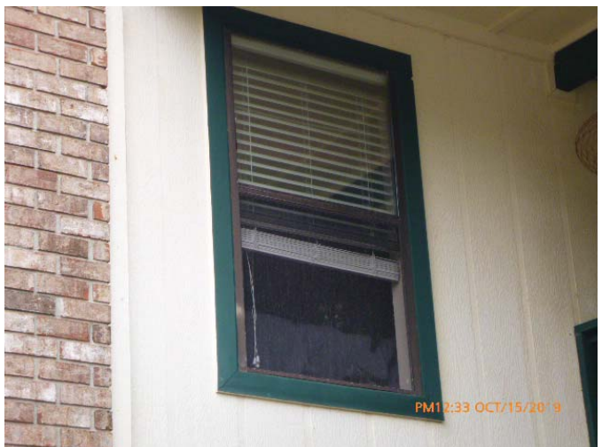
#7 - Opening Protection - None
