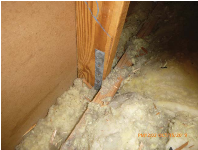
#4 - Roof to Wall Attachment - Hurricane Clips
