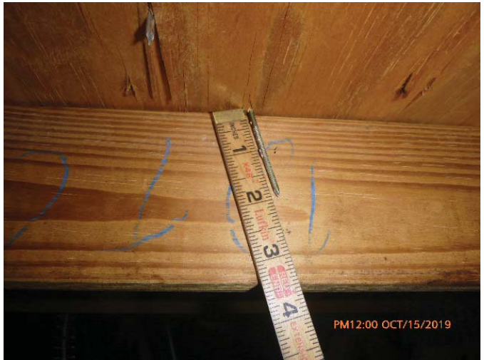
#3 - Roof Deck Attachment - 8d Nail
