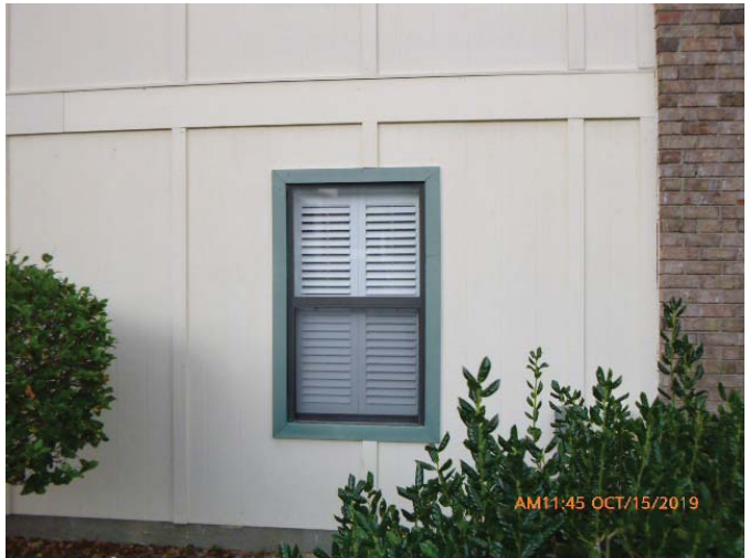
#7 - Opening Protection - None
