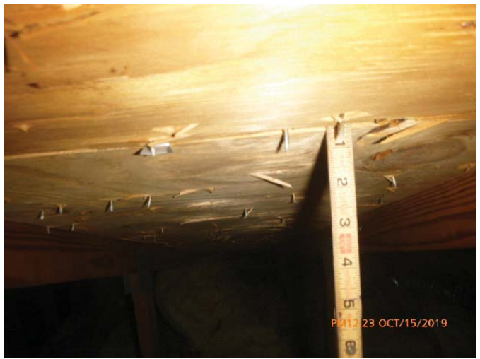
#3 - RDA - Sheathing Thickness 7/16" or Greater
