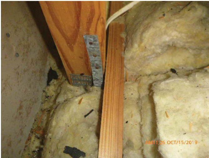
#4 - Roof to Wall Attachment - Hurricane Clips
